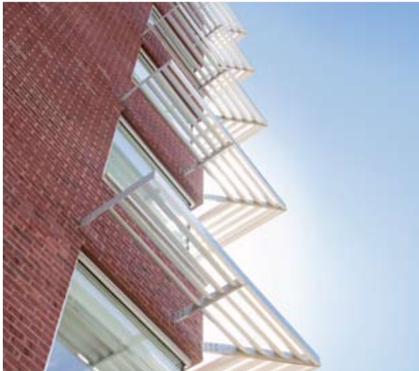
ABOVE Fox Point's exterior has attractive sun shades that limit heat absorption in the summer months. The building's walkways and floors use green material.
